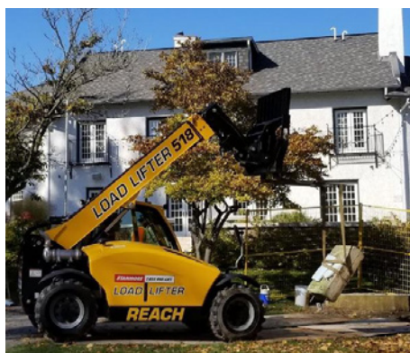
Installing the Queen Victoria Richmond Stone behind the restored Guild Inn, October, 2020.
